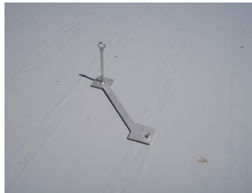
Fig. 2: Arrangement of the base feet
