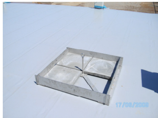
Fig. 8: Insertion of the concrete flagstones
