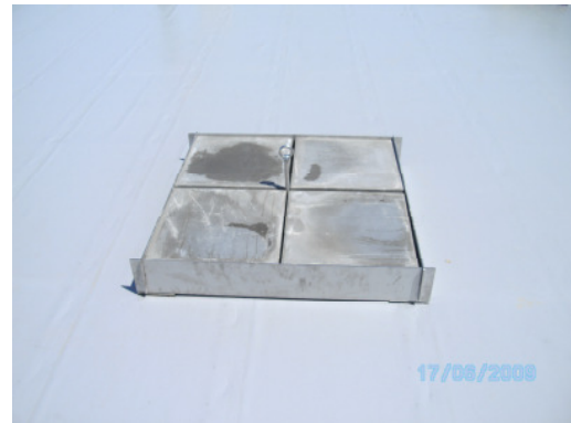
Fig. 9: Completely filled bordering
