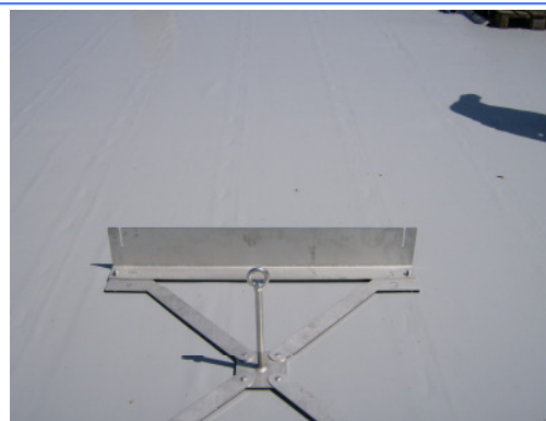
Fig. 4: Installation of the bordering
