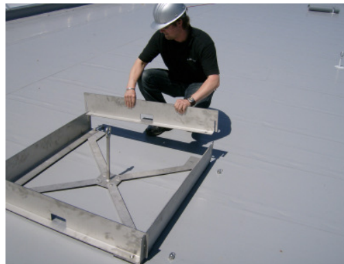
Fig. 5: Insertion of the upper side parts
