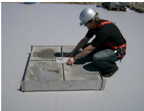
Fig. 10: Installation of the load distribution plate
